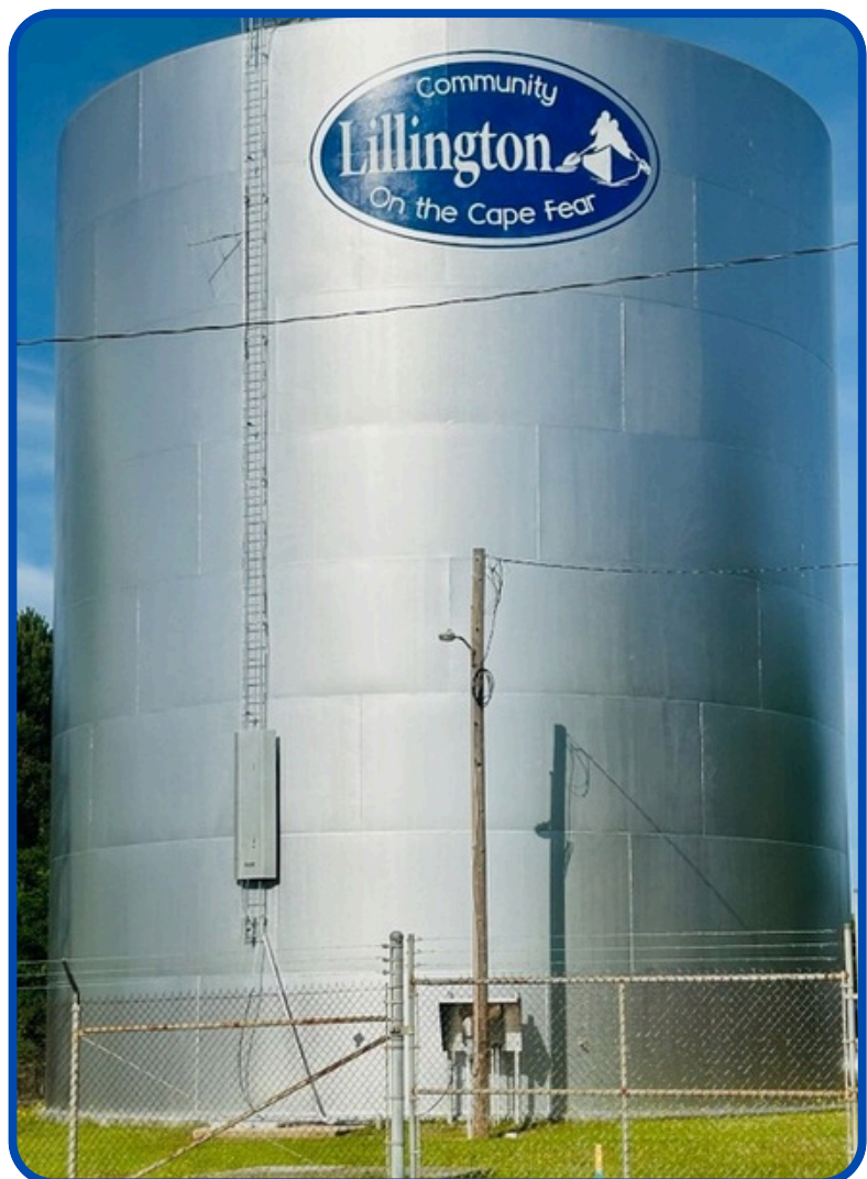
Town of Lillington ground-level water tank
