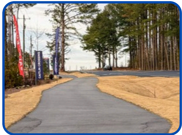
Newly constructed paved sidepath along Matthews Road
