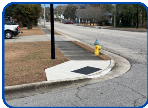
New curb ramp at an intersection.
