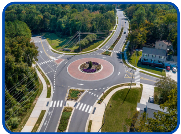
Town of Cary new roundabout.
